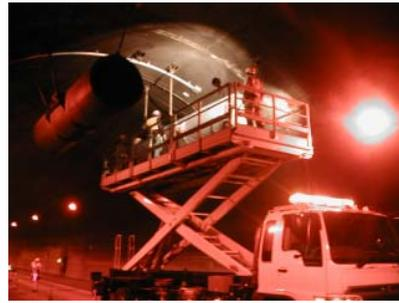
Fig. 2 Installation of the sensors to the jet fan
